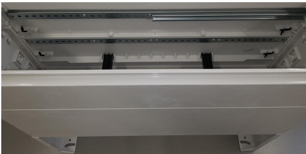
Figure 5-8 Installation of the C-profile rail (for the cable clamps)
