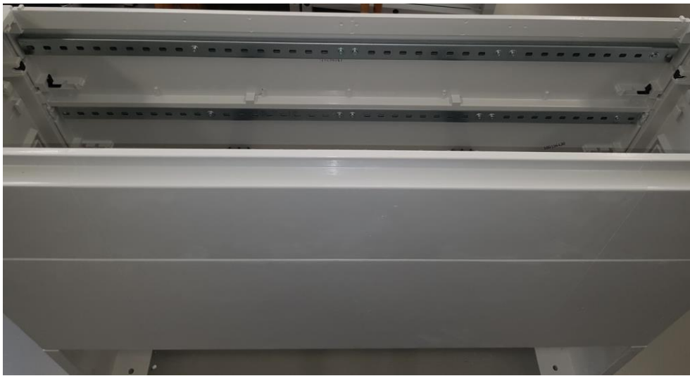
Figure 5-7 installation of the C-profile rails
