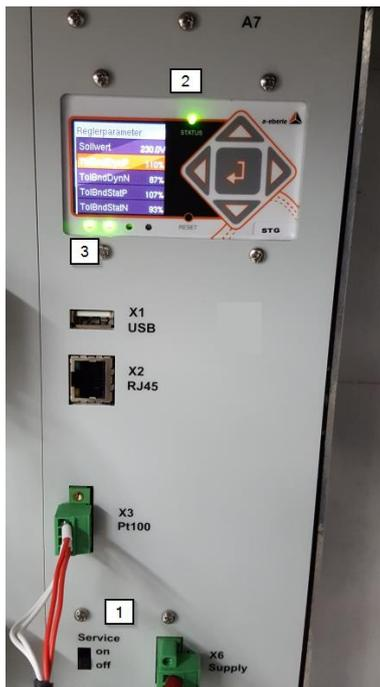
Figure 9-2: Slide switch service / lamp status
