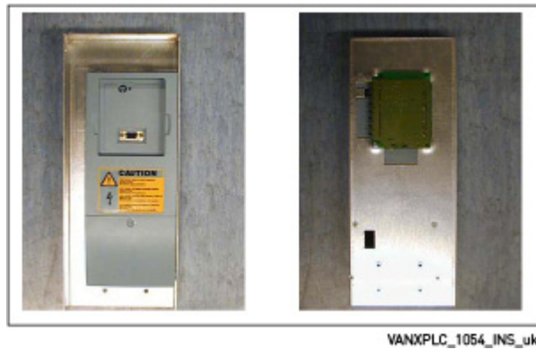
Figure 17. Control unit installed into the mounting box; Left: front; Right: back
