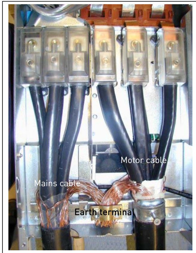
Figure 6-18. Cable installation in Vacon NXS/P, FR8
